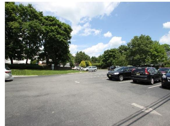
Rainwater on the site drains onto the road. The parking spots east of the building can be replaced with porous asphalt to capture runoff. There is also an opportunity for a rain garden to be installed north of the building to capture roof runoff. A preliminary soil assessment suggests that soils have suitable drainage characteristics for green infrastructure.
