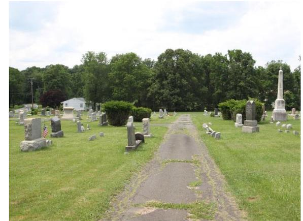
Rainwater from the church parking lot drains onto the road. A rain garden could be built south of the lot to capture, treat, and infiltrate runoff. Additionally, the cracked paved walkway in the cemetery could be replaced with porous asphalt to allow water to infiltrate. A preliminary soil assessment suggests that the soils have suitable drainage characteristics for green infrastructure.
